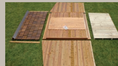
2. LAY OUT PRE-MADE PANELS
